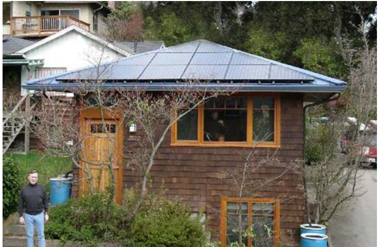
PHOTO CREDIT: PUGET SOUND SOLAR
